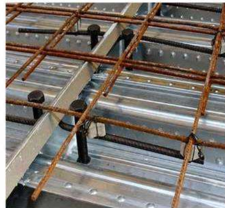
Figure 6. Demountable shear connectors with partial depth edge trim and U-bars
