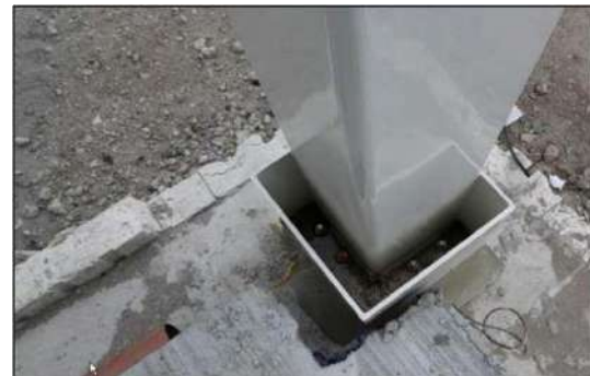
Figure 8. Shield plate to keep base plate connection accessible after concreting
