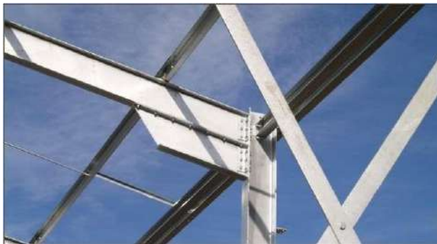
Figure 7. Bolted haunch plate connection
